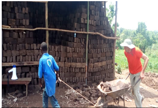
Richard (UK) working on the bricks project
